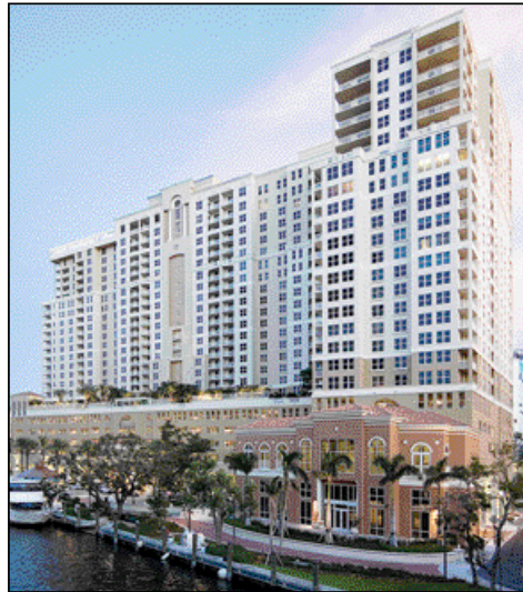
The 25-story, 409-unit NuRiver Landing luxury high-rise condominium situated on Fort Lauderdale's historic New River is in the area's trendy, downtown Las Olas area. The project was developed by Fort Lauderdale-based NobleHouse LLC and Washington, D.C.-based Carlyle Group. Photography by Nathan Selikoff and art direction by Lorraine Lax.
